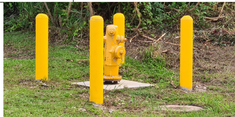
Installation of a New Fire Hydrant
