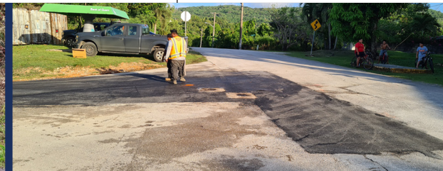
Pale Ferdinan Water Line Replacement Project
