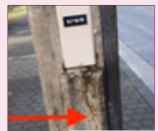
Tumon Streetlight Poles: Along with the other infrastructure installed in Tumon Bay Infrastructure and Beautification Project (TBIB), the street lighting and crosswalks systems (below) are now approaching 23 and 19 years of service in Phase I and Phase II, respectively. Since their initial installation, the crosswalks and streetlighting system have been and are subject to the wear and tear of traffic and time.
