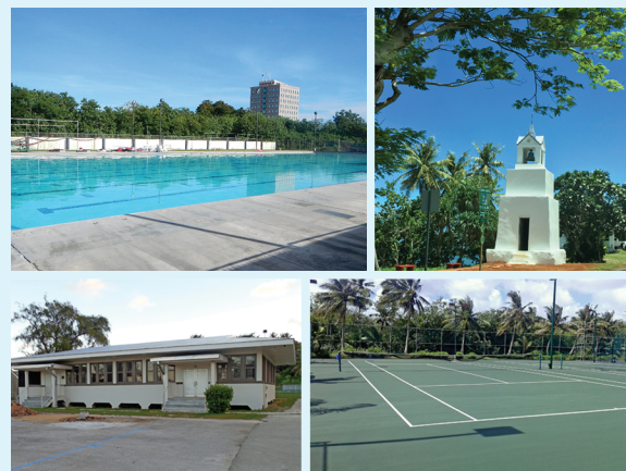
Hot Bond Completed Projects: Hagåtña Swimming Pool, Malesso Bell Tower, Inarajan Community Center, Hagåtña Tennis Facility
